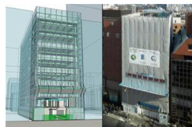
BIM model visualizing the construction and the site photo
